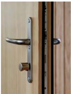
The exterior doors in a Passivhaus are thicker than a regular door and seal to their frame for thermal and acoustic insulation. They are an integral part of the airtight building envelope.
