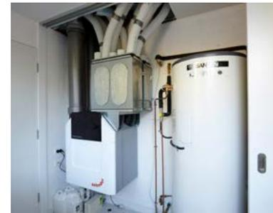
The mechanical ventilation system with heat recovery (MVHR) for a single-family home is typically only the size of a clothes dryer and is often installed in a cupboard in the laundry or hallway. The ducting is concealed in the ceiling with small vents in each room. The system is very quiet and uses less energy than a 50w halogen light bulb.
