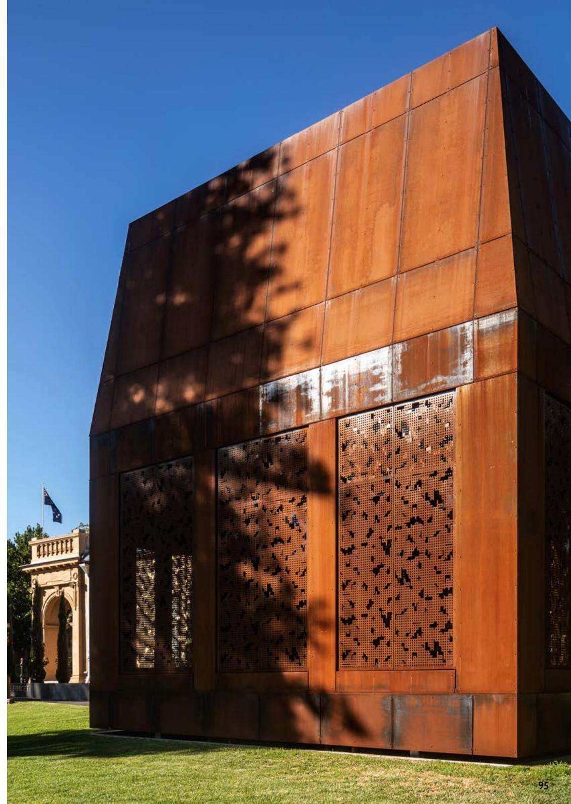
Maintaining a AA-standard environment for both the gallery and storage spaces could have made for expensive running costs. However the chosen combination of high levels of insulation, an airtight envelope and an energy recovery ventilation system have produced a highly energy-efficient building, slashing operational costs for mechanical systems and delivering a space that is very comfortable to occupy.
